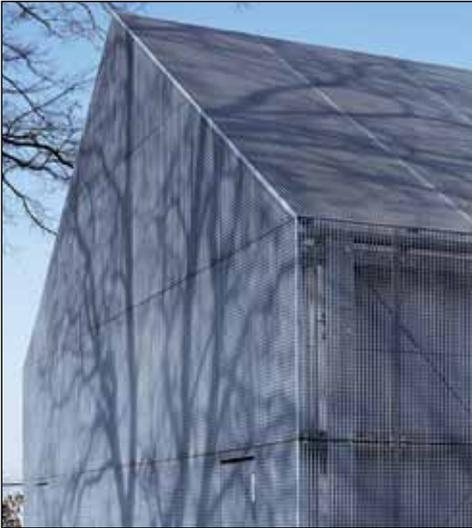
**4** Aluminium-Fassade mit feuerverzinkter Tragkonstruktion
